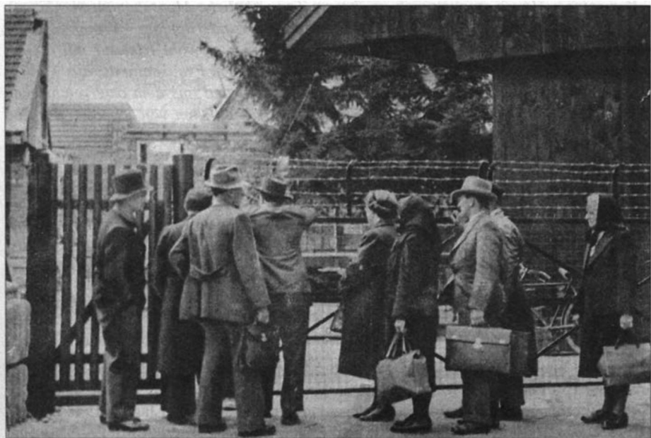
The front end of a queue in front of Irlmaier's property on Waldstrasse (today Jennerstrasse).
